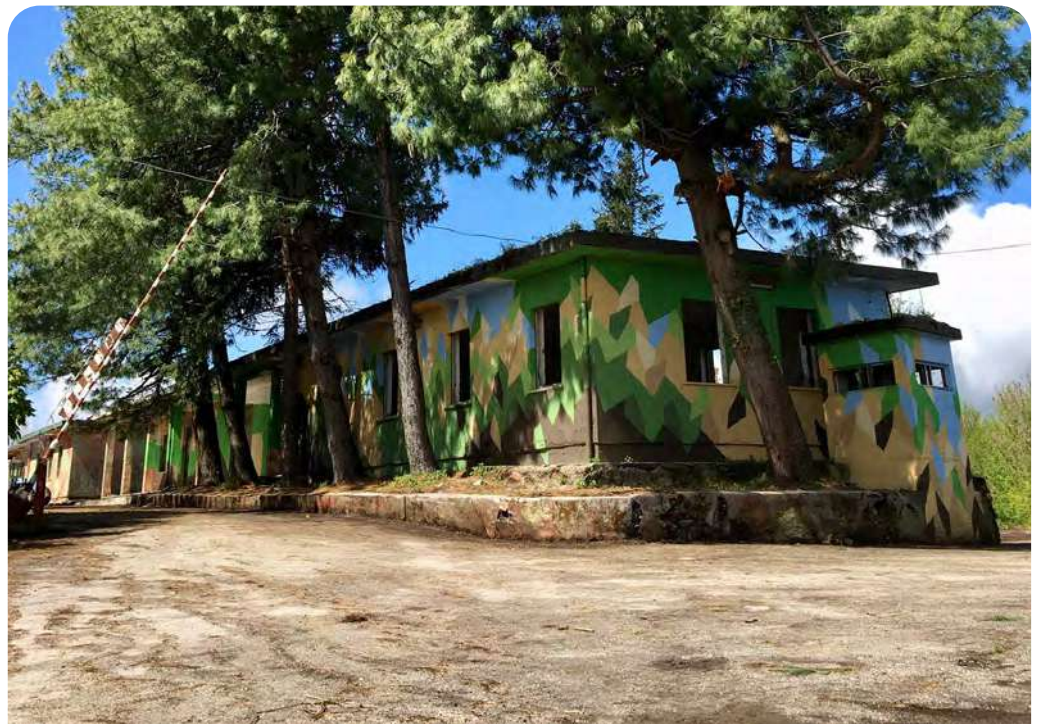
Former military base Calvarina, main building
